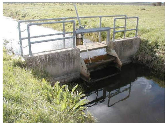
J. Older style tilting weir
