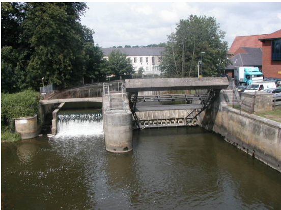
A. Radial gate, right.
