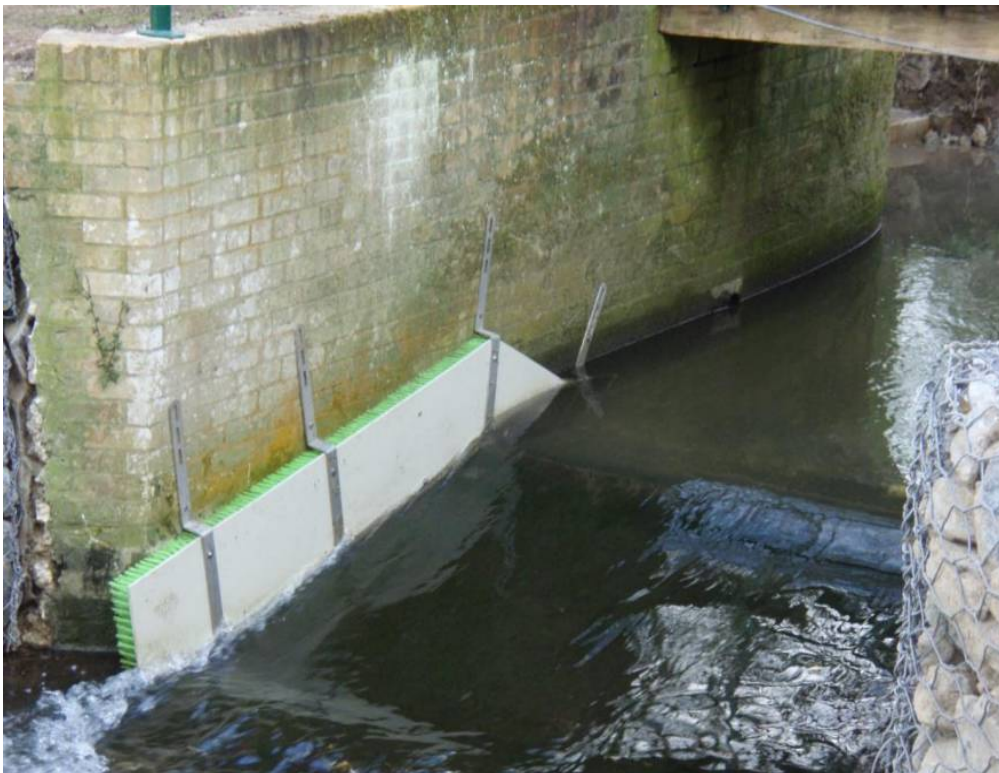
Figure 4.13: Installed pass, showing brackets and fixings
