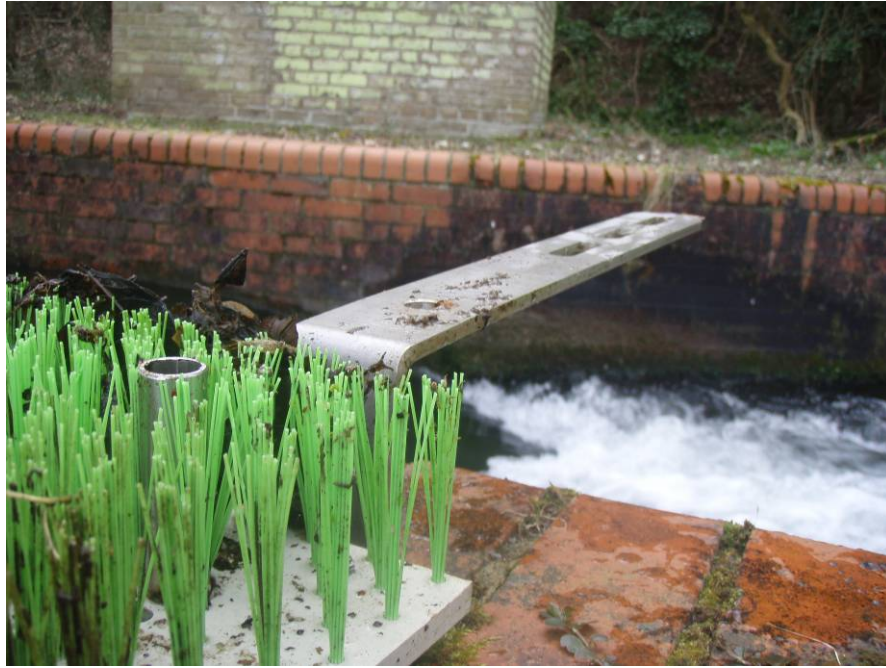
Figure 4.7: Stand-off bracket and spacer with board fixed
