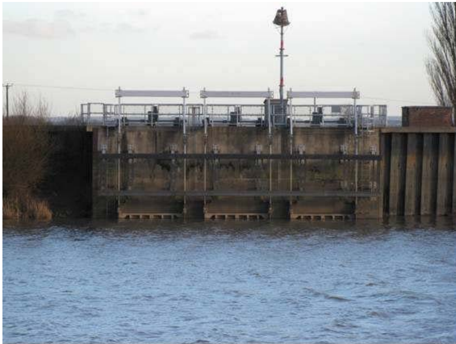
Figure 7.26: Counter-balanced gates on the Bottesford Beck, Scunthorpe.
