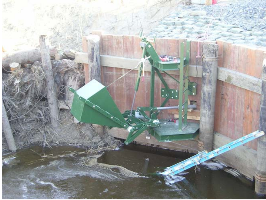
Figure 7.7: Float mechanism for an MTR gate at Schneider Creek, Washington State, US. Photograph courtesy of Tom Slocum, Washington Conservation District's North West Region Engineering Program.
