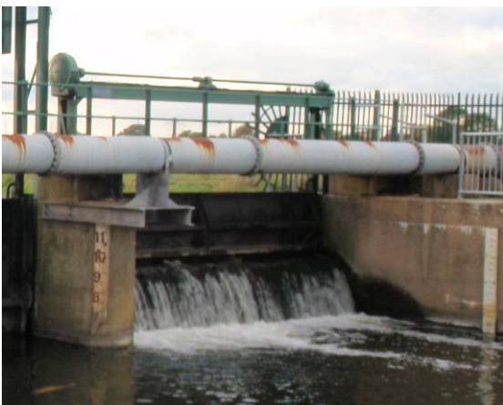
C. Small penstock sluice
