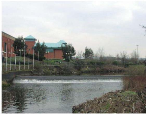
Figure 4.4 Rectangular Weir
