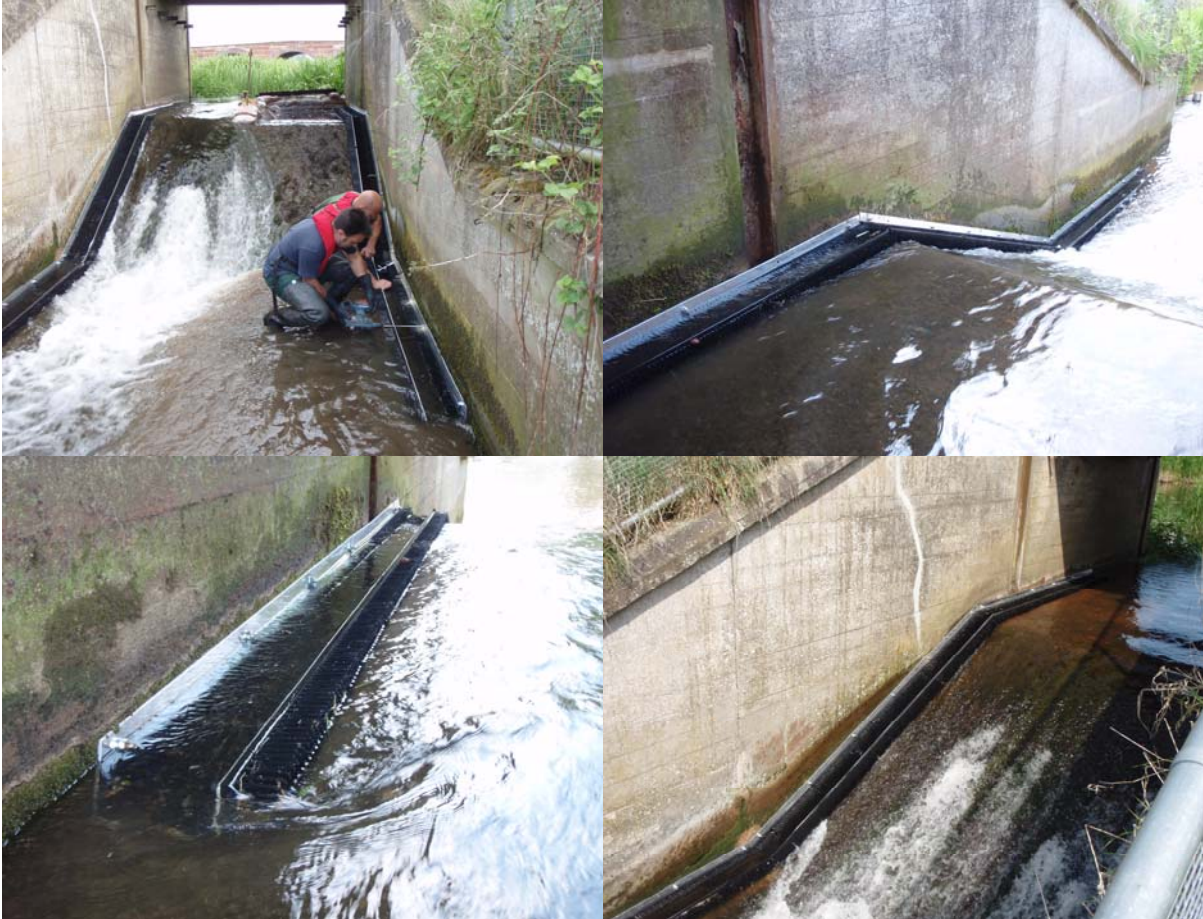
Eel pass at Stapleford Mill weir, on the River Gowy: under construction and completed.
