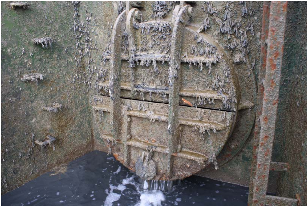
Figure 7.10: Tidal flap at Maydays Farm, Essex. This is an interesting installation as the flap is separately hinged in two halves. The lower half is fitted with a small 'cat-flap', presumably designed to operate at very low flows. However this cat flap, which is made of cast iron, is too heavy to make a useful contribution to elver passage.
