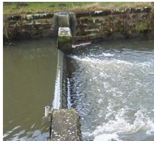
4. Contracted thin plate weir
