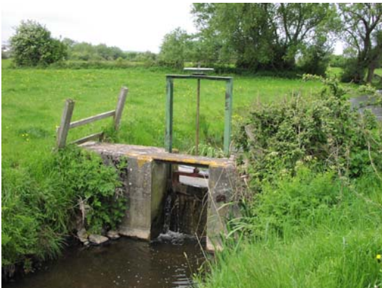
C. Small penstock sluice
