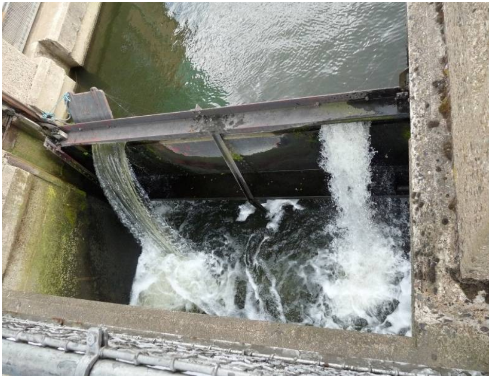
Figure 7.17: Two mouse holes on a tidal sluice on the River Medway.
