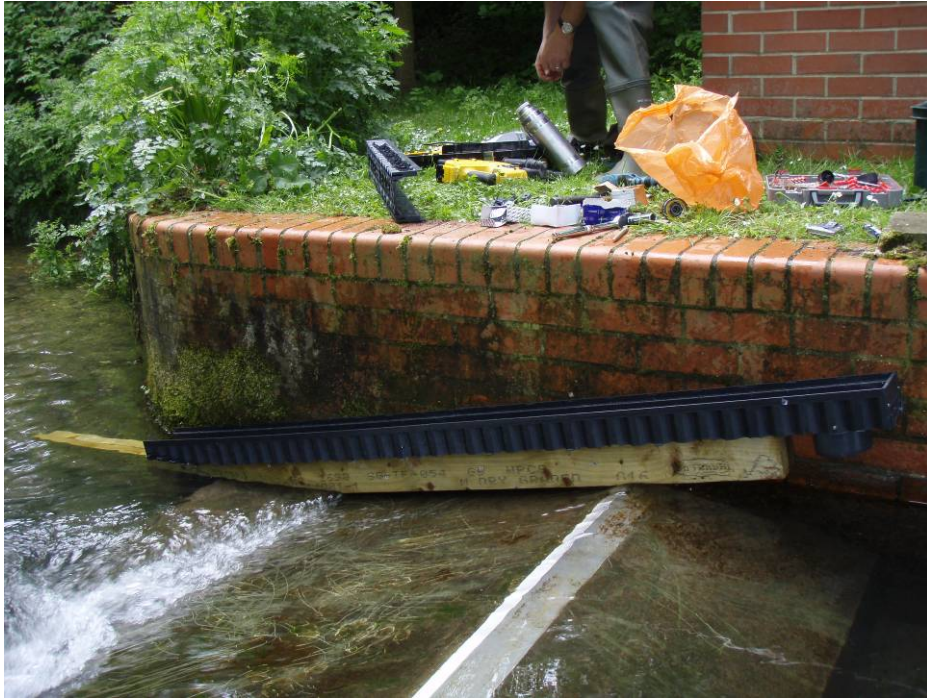
Figure 4.18: Crawling gutter under construction. These curved wing walls are found on many gauging structures. (Note the layer of fast-moving water on the downstream weir face and the clean, debris-free surface. Elvers and eels would be unable to swim through this structure.)
