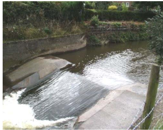
2. V Shaped broad crested weir
