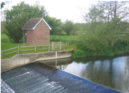
Figure 4.2 Single crump weir
