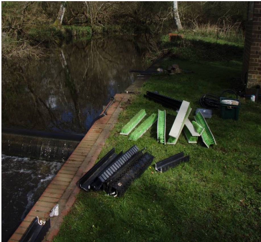
Figure 4.19: Gutter pass materials and bristle mat substrate being assembled on site.
