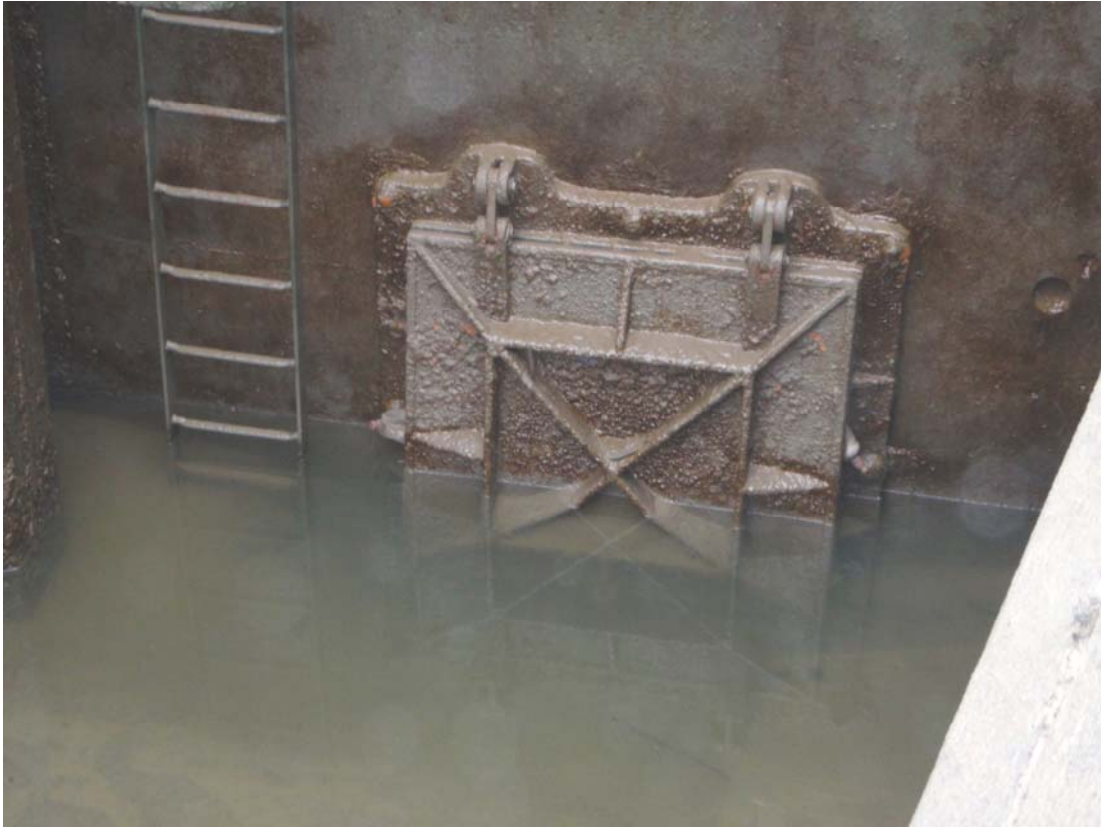
Figure 6.9: The outer flap in the structure shown in Figure 6.8. Note the two plastic bottles jammed in the flap which prevent the flap from closing completely. Were this a single flap, the jammed bottles would allow some landward flow and the passage of elvers. However, the presence of a second flap a couple of metres behind this one prevents this.
