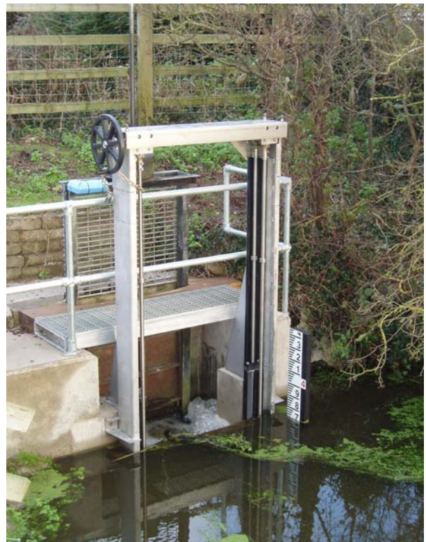
D. Twin leaf gate (above) E. Large undershot gate (left)
