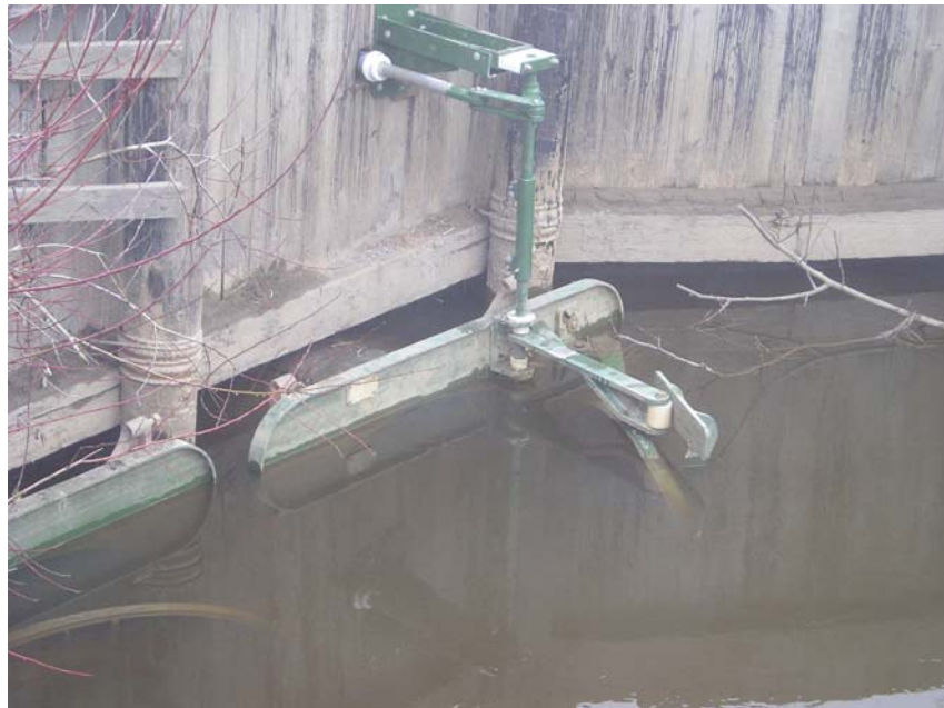
Figure 7.8: Gate actuating mechanism for an MTR gate at Schneider Creek, Washington State, US. The door is being held open. Photograph courtesy of Tom Slocum, Washington Conservation District's North West Region Engineering Program.
