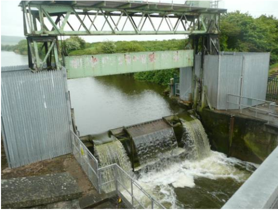
F. Penning weir (door down)
