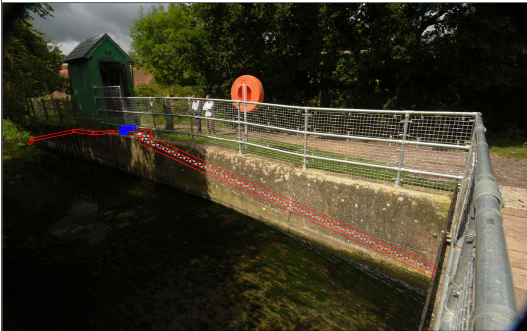
Figure 8.1: The route of a typical downstream channel with substrate, the flow splitter box (blue) and the upstream delivery pipe (red).
